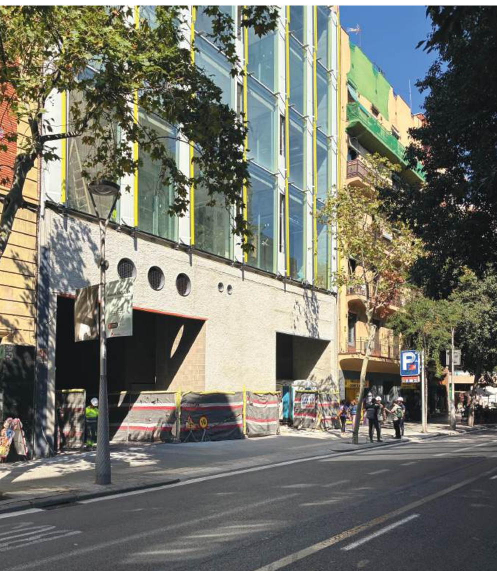
New Facility - Mallorca St. facade under construction October 2025
