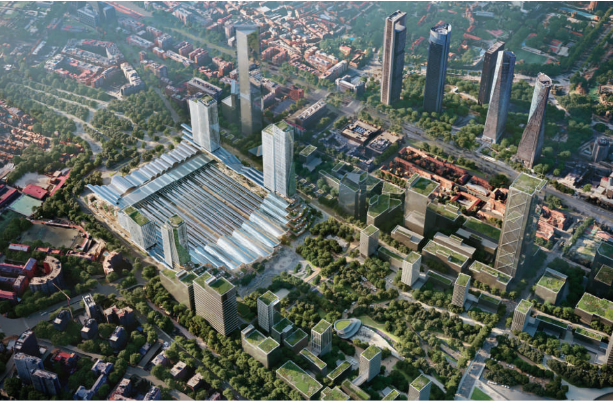
Chamartín-Clara Campoamor Station will be the core of the new mobility system, fully integrated into the city grid. Source: Adif.
