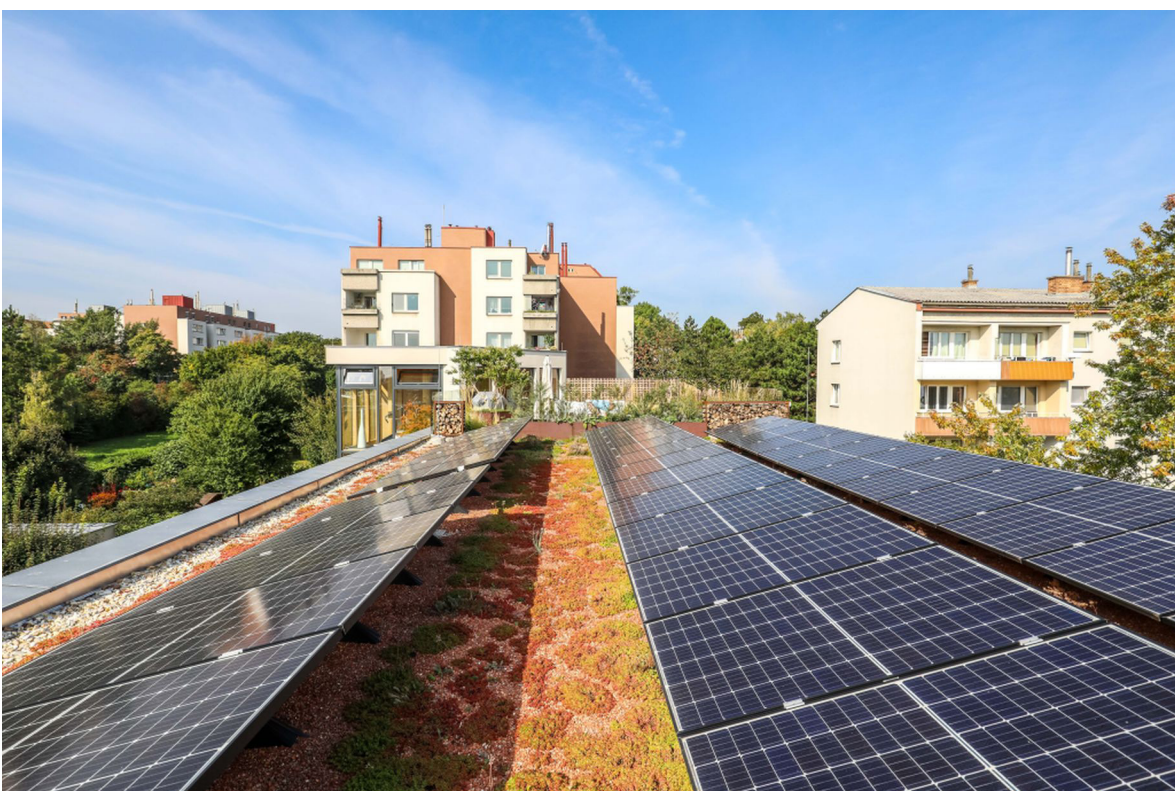
Planning for the Energy Transition Copyright StadtWien ChristianFürthner
