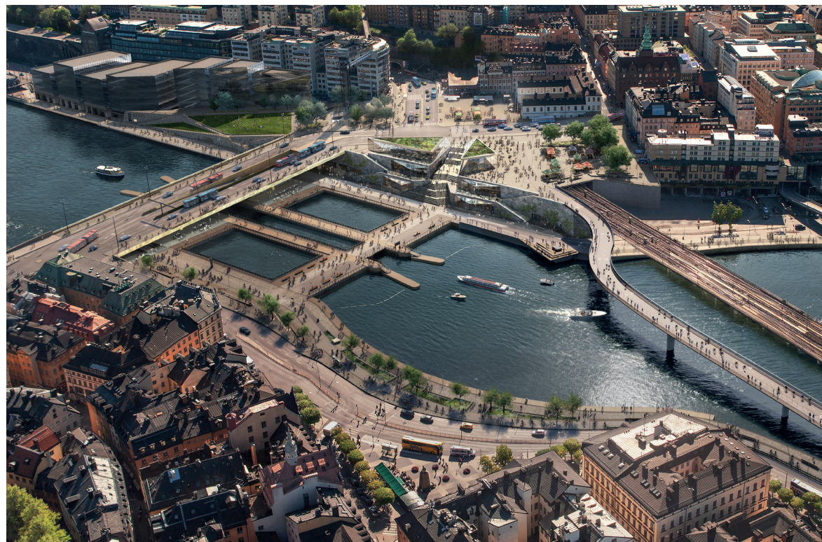
SLUSSEN – public space, transportation hub, water discharge technical system.
